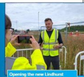
Opening the new Lindhurst Spine Road that unlocks a £250m investment in Mansfield
